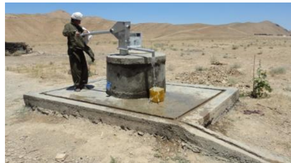
Fig 14 – Completed new well with drainage curtain
