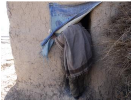
Fig 19 – Demonstration latrine with internal wall and plastic sheet door
