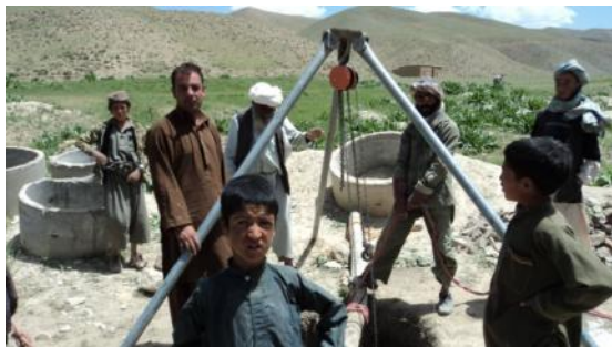
Fig 11 – Well under construction
