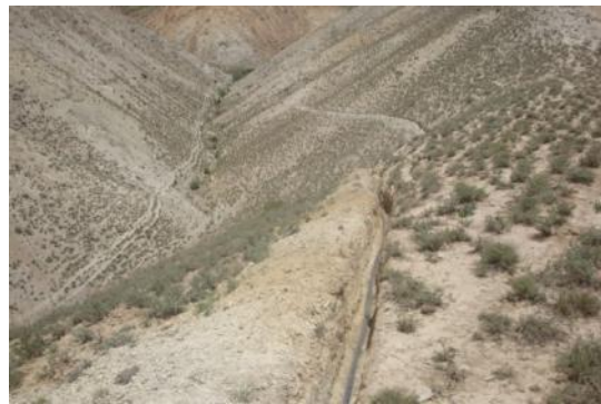
Fig 16 – Pipeline dug for gravity supply
