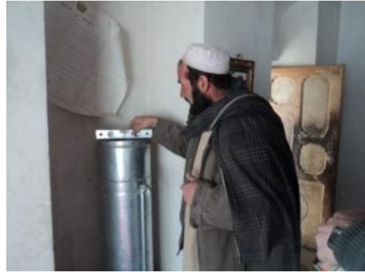
Fig 10 – Levelling the biosand filter during installation
