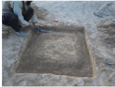
Fig 18 – Training on constructing the modified 'square' domed slab
