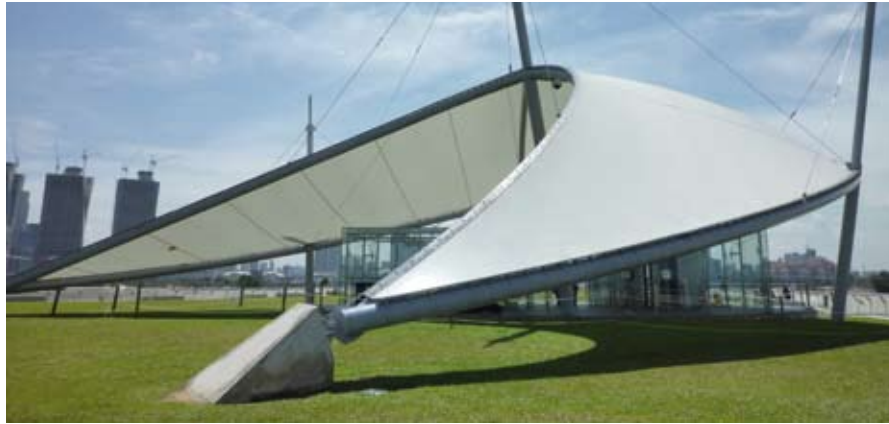
Marina Barrage green roof
