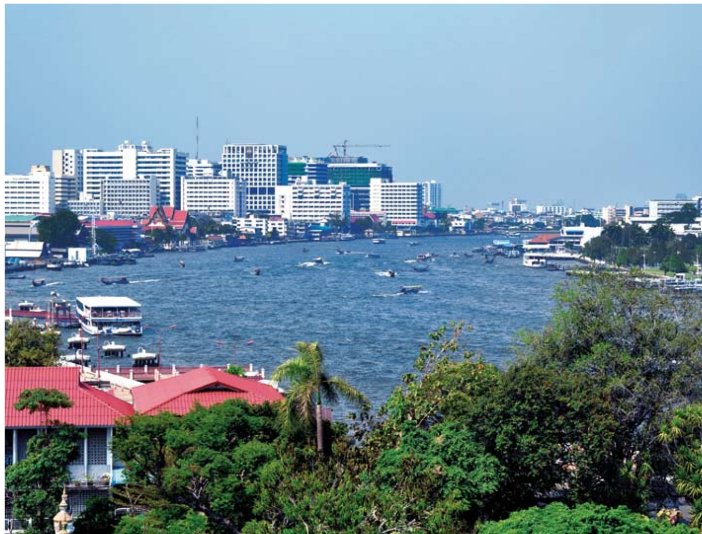
The human settlements designed and built in adaptation to waterscape proved their resilience by withstanding the disastrous floods
